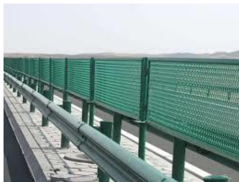
Figure.1.2 The W-beam and the pillar structures of highway fence.
